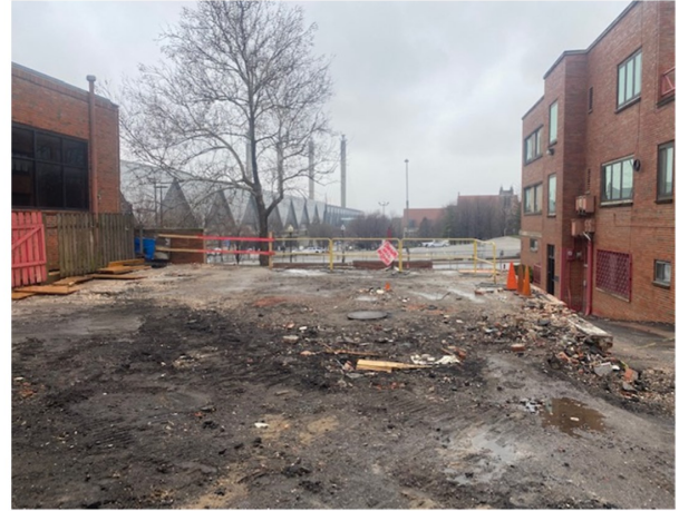
Garage Demolition Footprint
